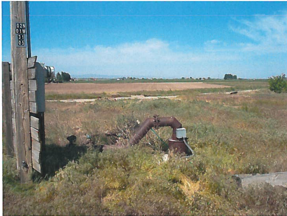
63-11739 Exam 5/16/2012: POD facing west. Canal, ditch, and dirt road between canal and ditch in photo middle-ground. Portion of POU on other side of canal in photo background.
