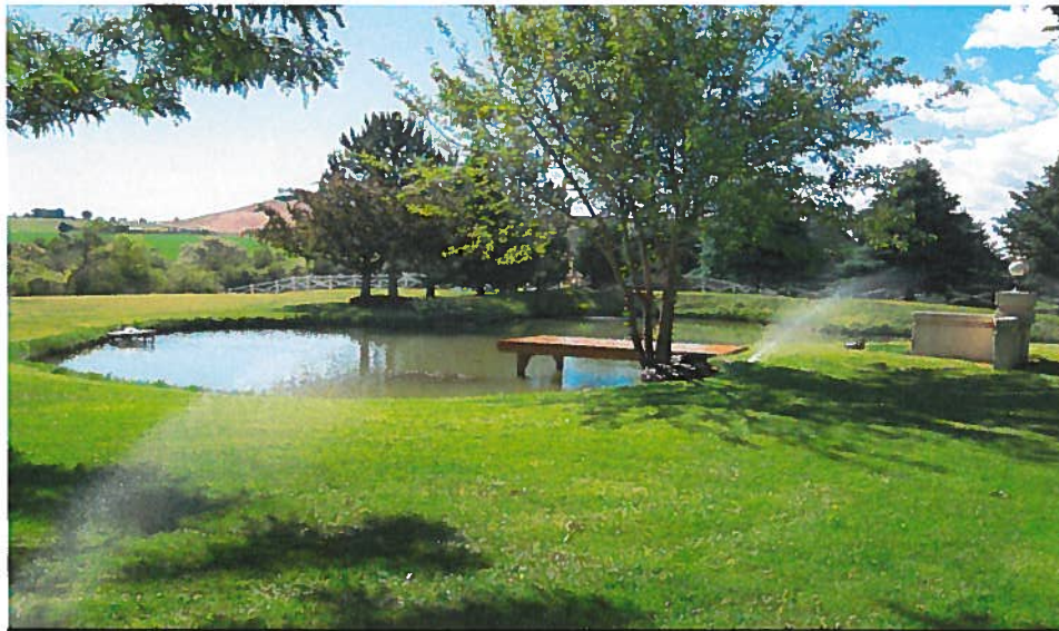
View southeasterly of irrigation pond and lawn sprinklers in operation. The bubbler platform for the river sewage pump discharge line is shown to the left.
