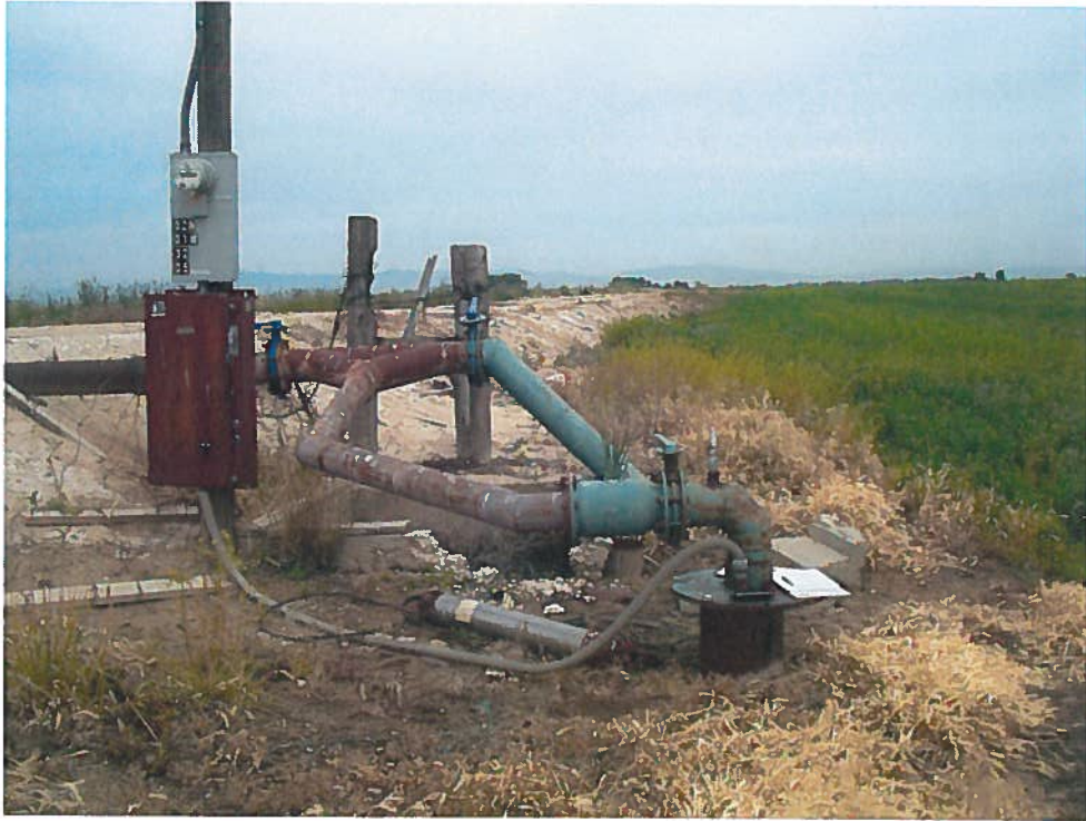
63-11682 Exam 5/15/2012: POD facing east. Green pipe is 8" mainline southeast to large pivot. Rust colored pipe is 8" mainline northwest cross/under canal to small pivot.
