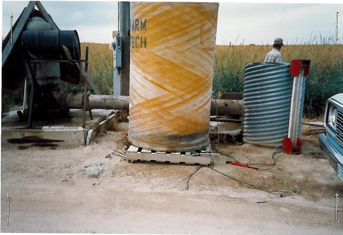
Well #3 Looking west.
