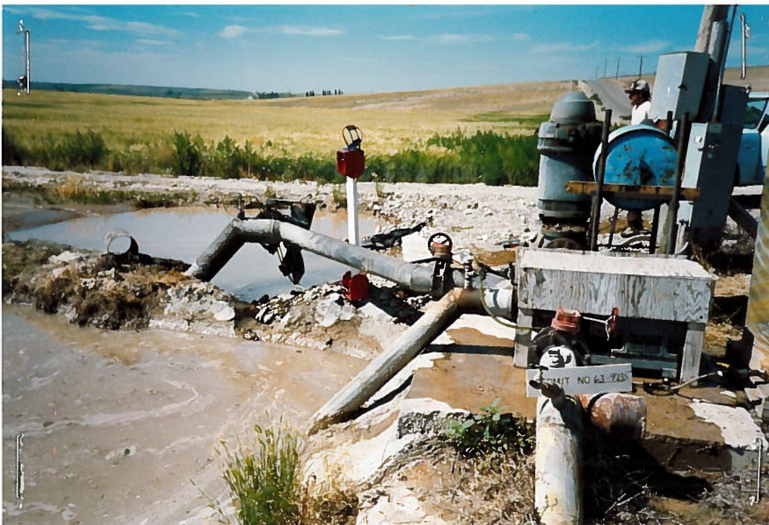
Well #4 Looking north P.U. in back-ground. Note: the permit sign reads 63-9735 because at the time of the examination I was told that this well was the PP p.d. for that permit. photo taken 6-26-87
