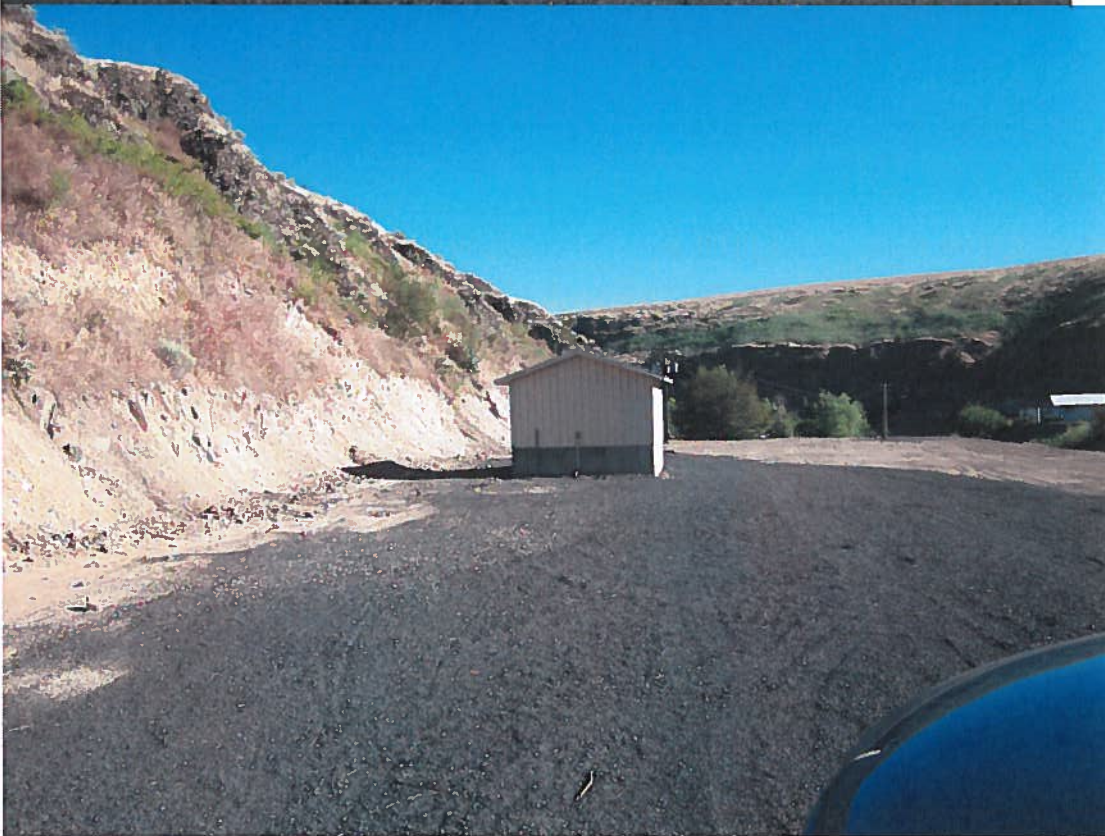
NORTH WELL HOUSE
