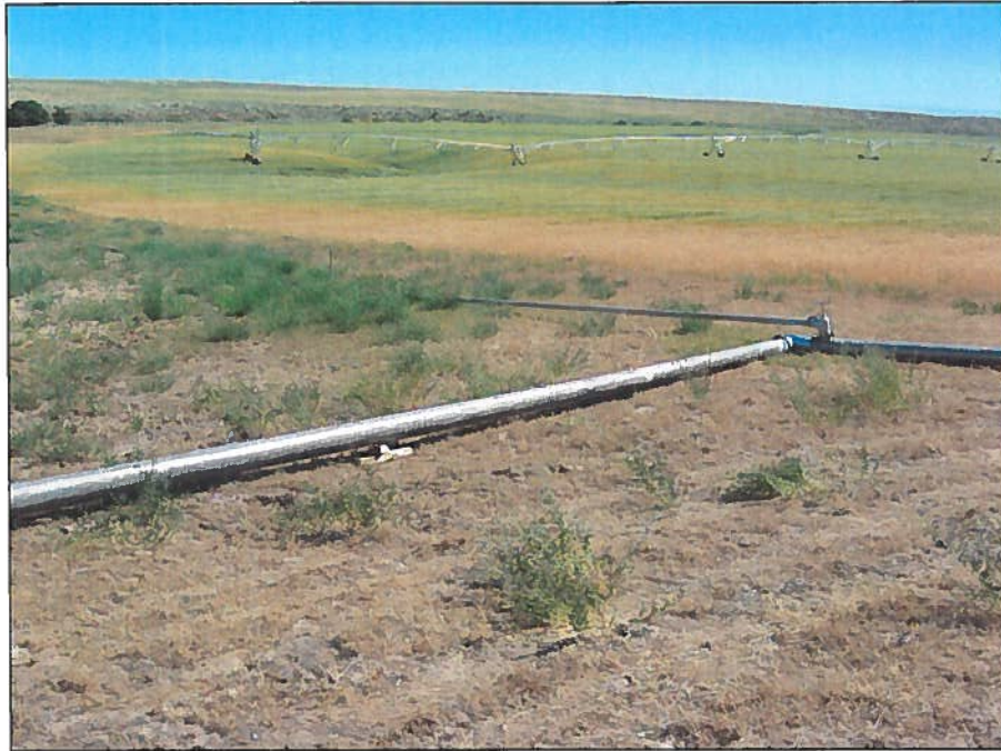
Photo 5: Aluminum mainline supplying handlines. Pivot #2 in background.
