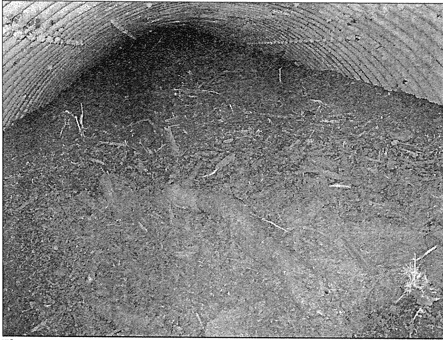
Figure 9. —Interior of Parks Creek culvert.
