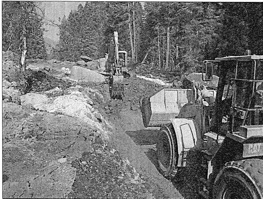
Figure 8. —Opening the road at Parks Creek, Site 8.
