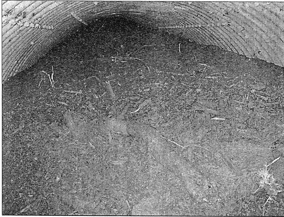
Figure 9. —Interior of Parks Creek culvert.
