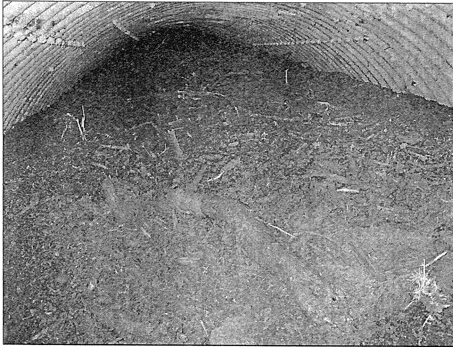
Figure 9. —Interior of Parks Creek culvert.
