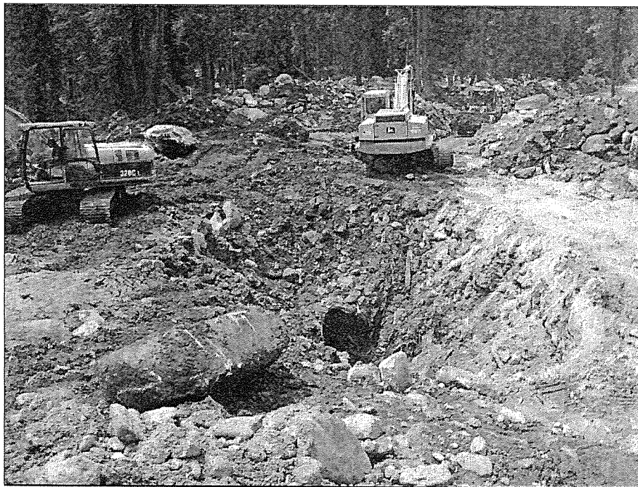
Figure 10. —Opening the Road at Parks Creek culvert (inlet shown).
