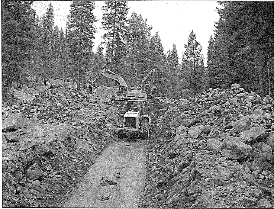
Figure 11. —Opening the Road at Parks Creek culvert showing road west of Parks Creek.
