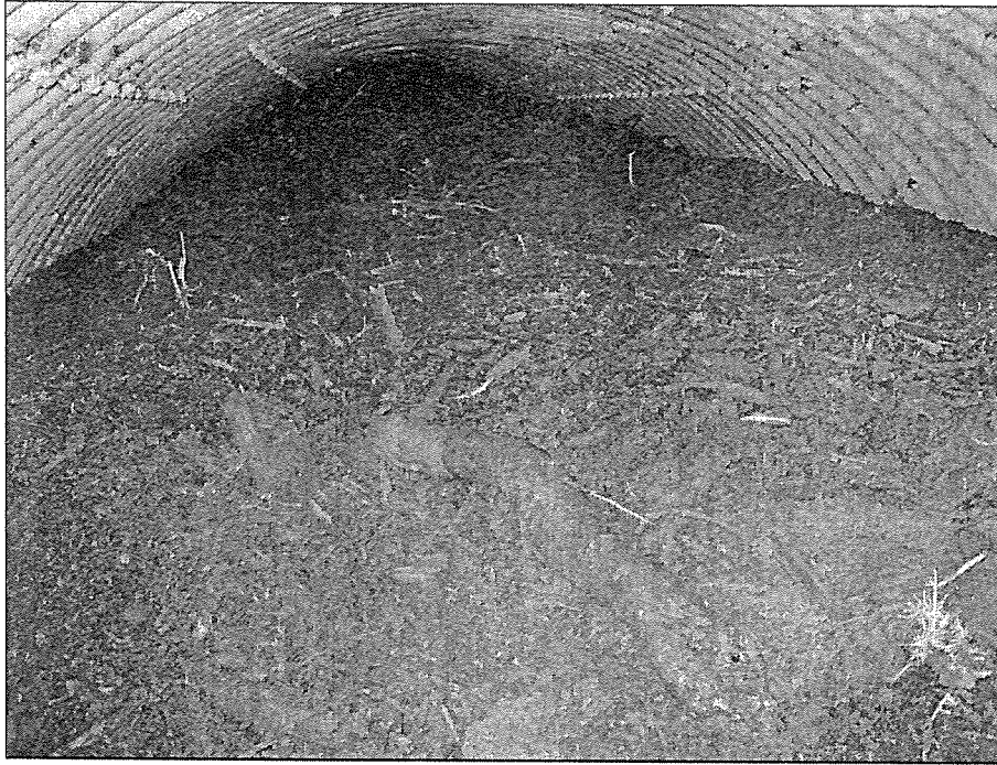
Figure 9. —Interior of Parks Creek culvert.
