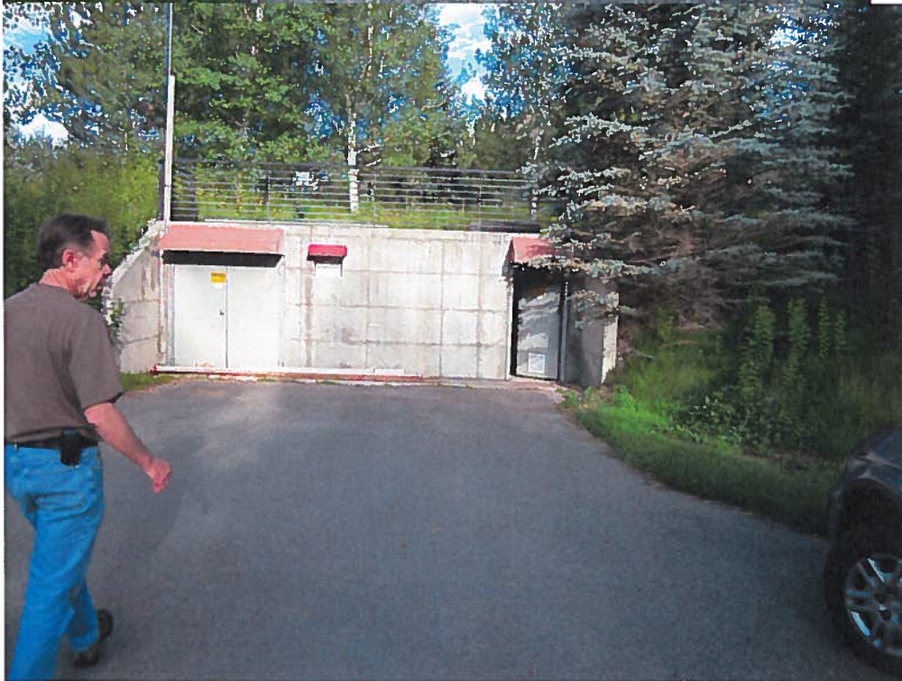
Pump House Facing W
