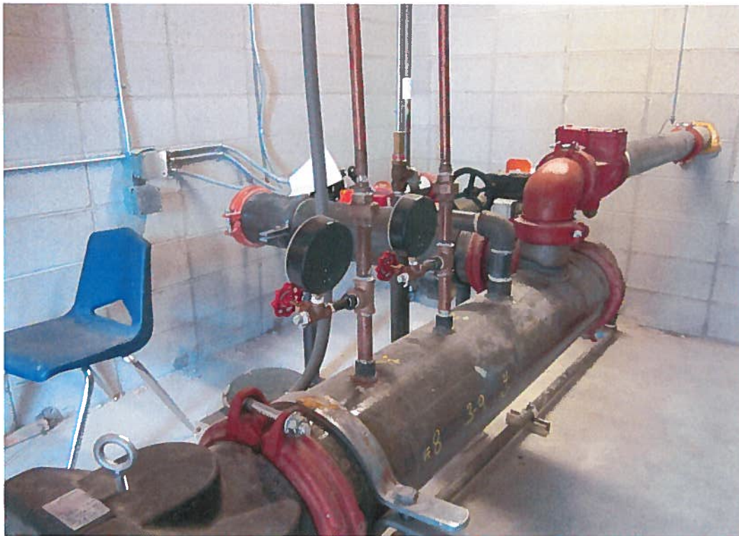
Riser room on north end of gym building. Water pipe to main building – middle left of photo.
