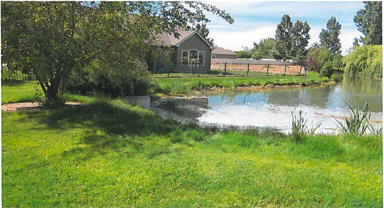
Point of Diversion/Place of Use: View northwesterly of Pond No.5. Concrete structure to the left is the pond system overflow structure. The overflow structure discharges into another concrete structure between Pond No.4 and Pond No.5, which discharges the pond overflow through a 12" diameter pipe to Ten Mile Creek.
