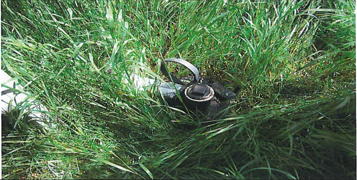
Point of Diversion: Ground Water well located in landscape next to Pond No.1. Well runs continuously to maintain pond levels and movement of water for the interconnected ponds.
