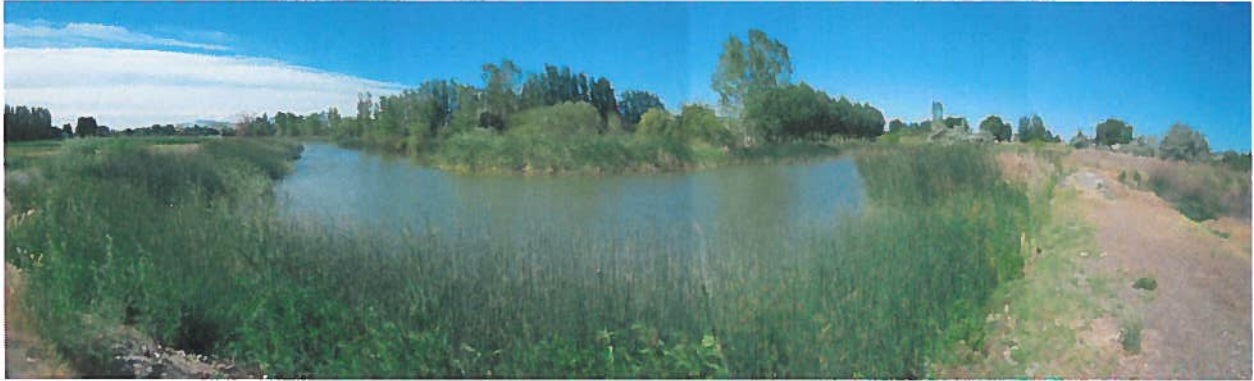
Photo of the pond from the northeast corner looking southwesterly. Gravel dike road on right side of picture.
