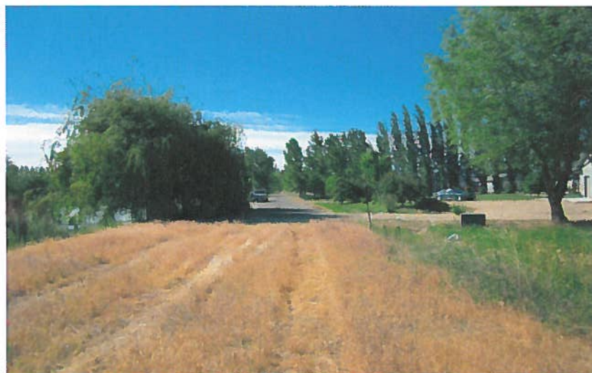
Dirt ditch travels along right side of access road
