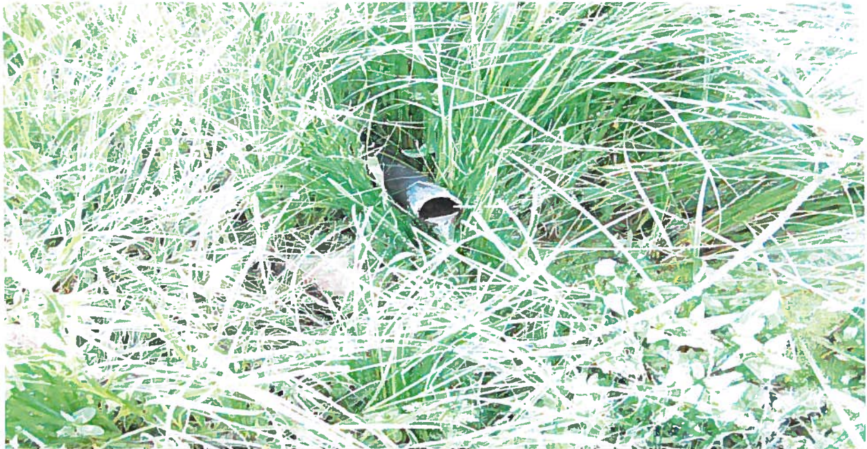
Place of Use: Stock water storage pond 2" PVC pipe supply line from spring box on neighbors property.
