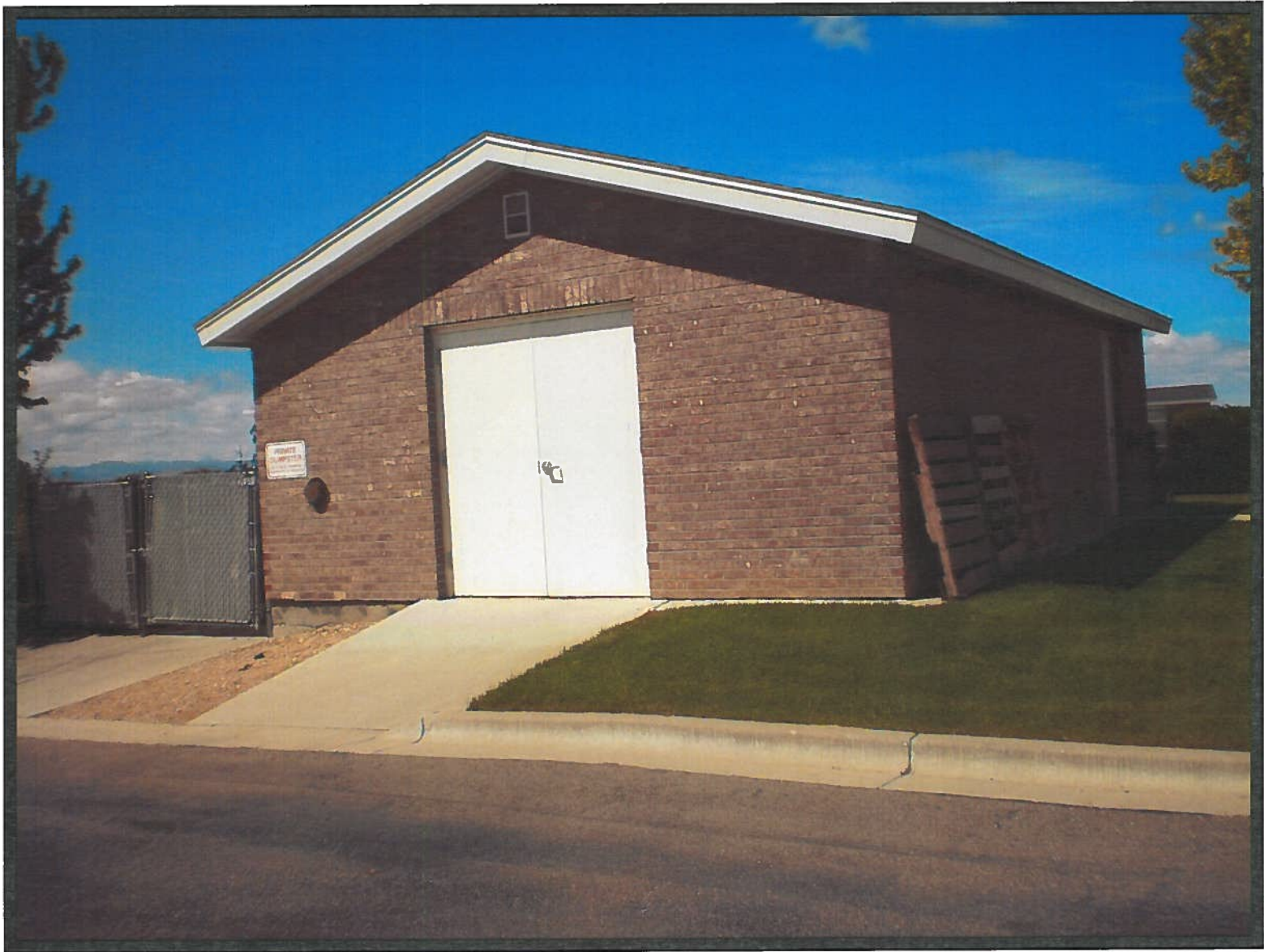
Well and pump house
