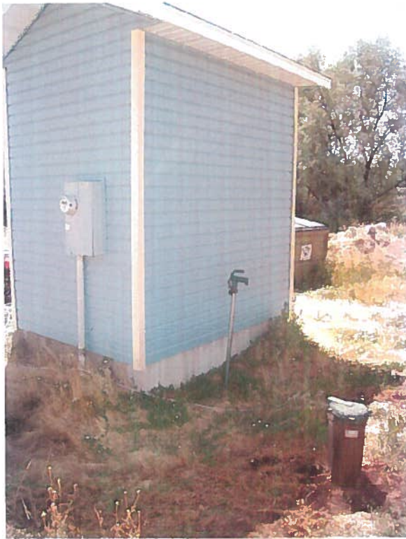
Pump house for four homes
