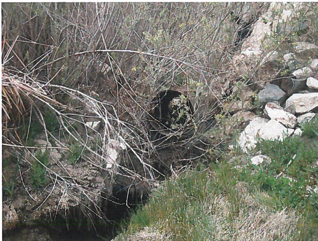
Figure 2: Outlet Pipe in Holt Creek Channel
