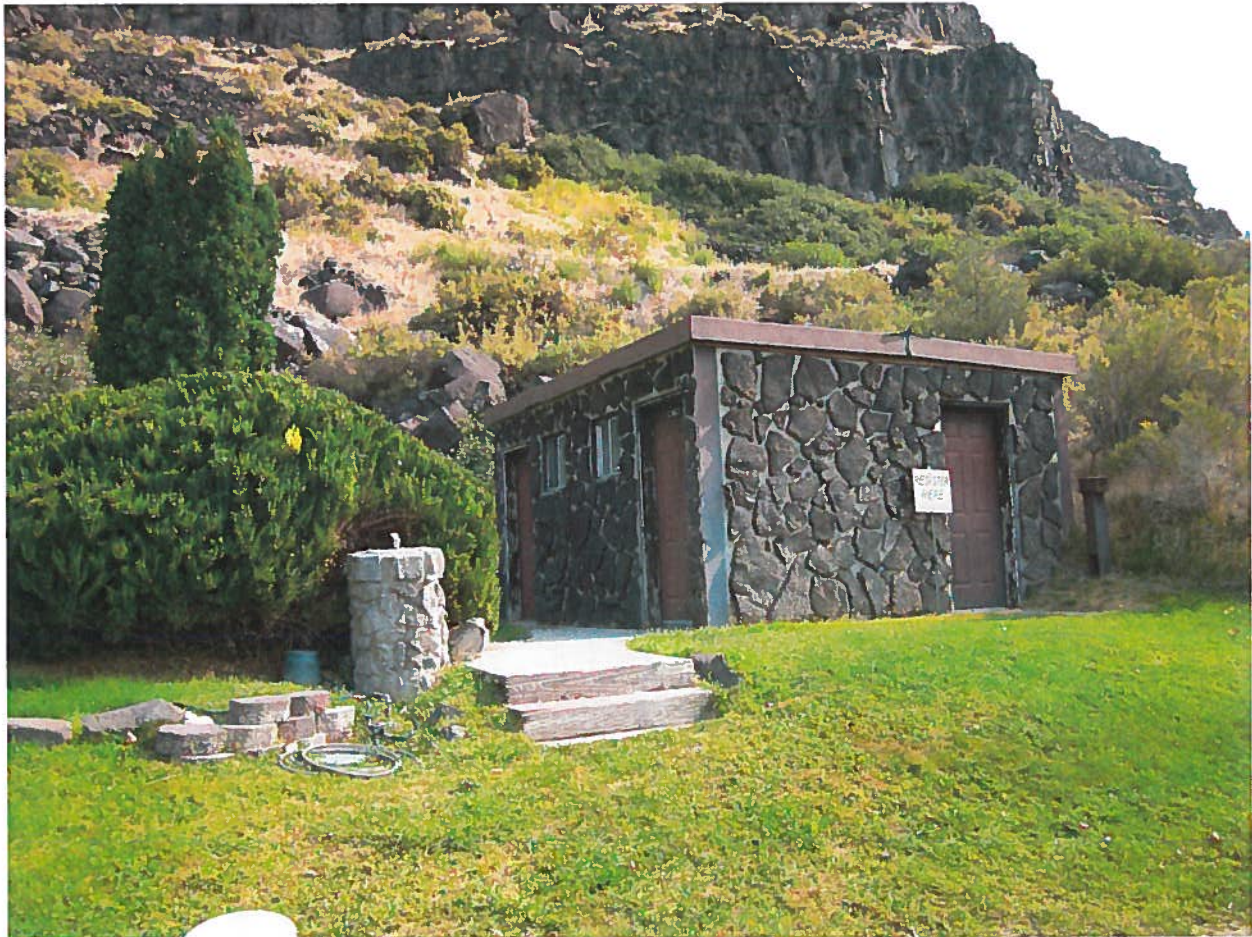
Figure 1: Restrooms and fountain
