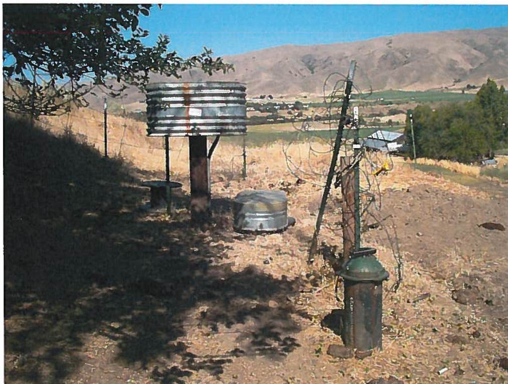
65-13831 Exam 7/30/2012: POD facing west. Well in foreground. Control box underneath upside down stockwater trough southwest of well.
