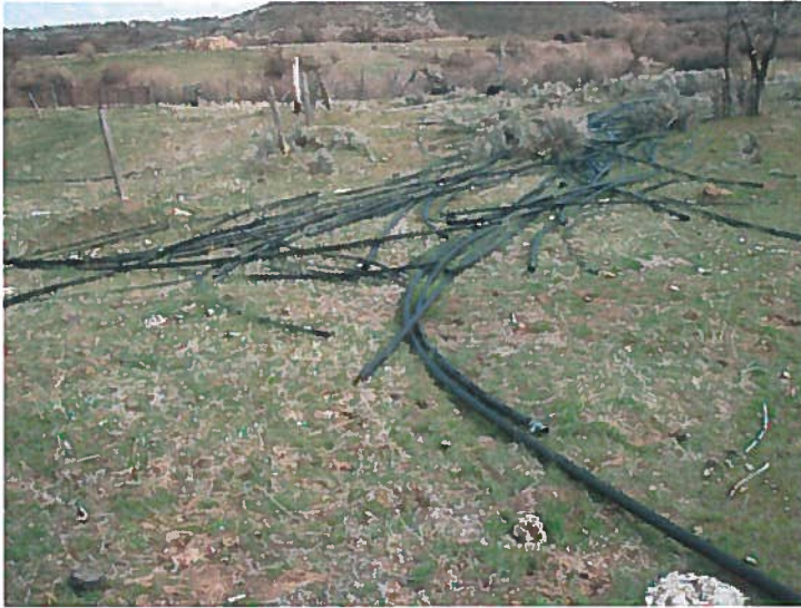
Figure 1: Polypipe used in the irrigation system. Located on the NE edge of the property.
