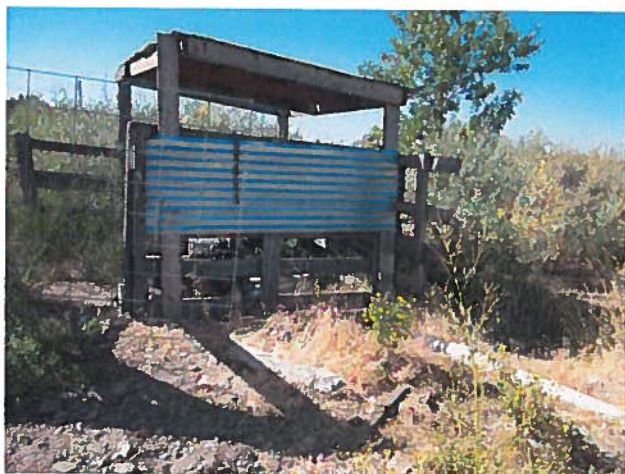
Pump house (POD)
