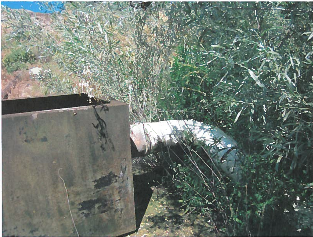
Excess water in tank flows back into Snake River.
