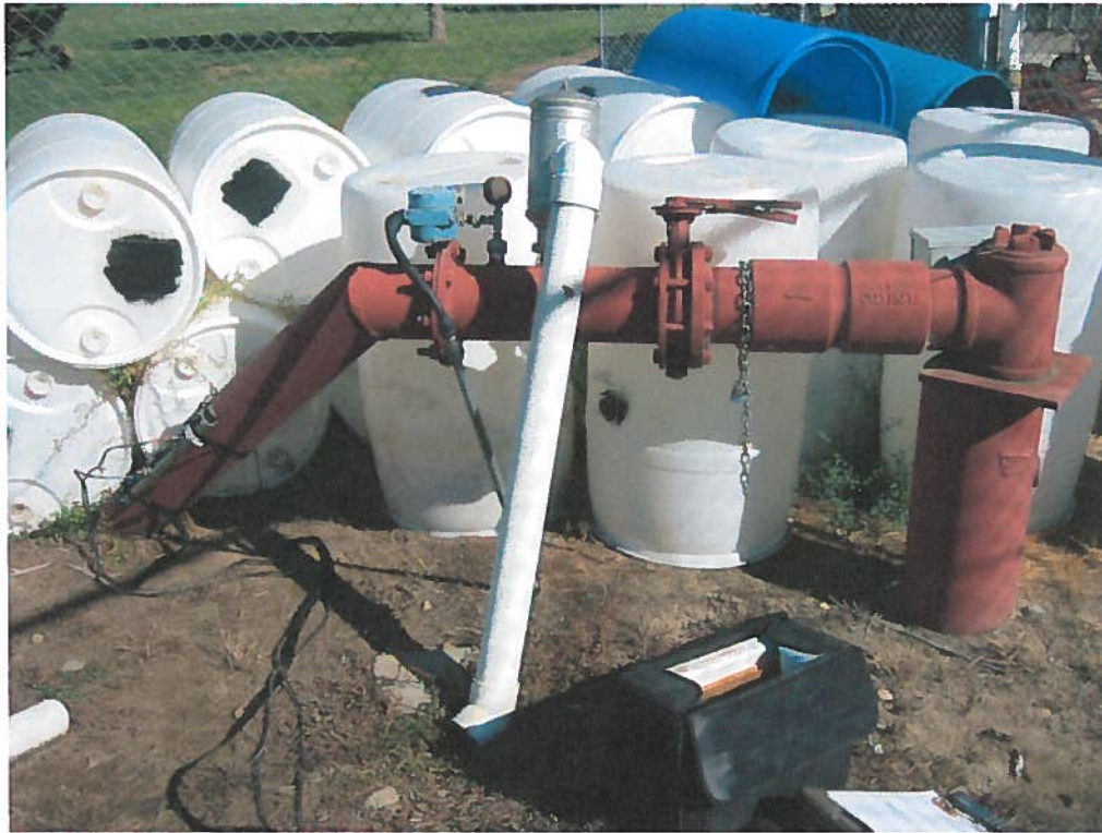
Photograph of irrigation well. Blue butterfly valve causing turbulent and messing up Thyme Flyte reading.
