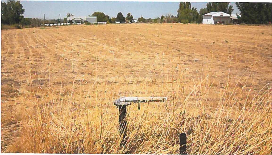
Diverter – Continuing west on Grandview Road from the above picture, looking north at the diverter for the irrigation system approximately 110 feet west of the first riser pipe.
