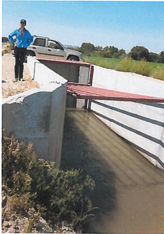
Licensed POD (also the permitted POD farthest from the POU) – Looking west along the waste water ditch and Grandview Road showing the new concrete sharp-crested weir at the licensed POD.
