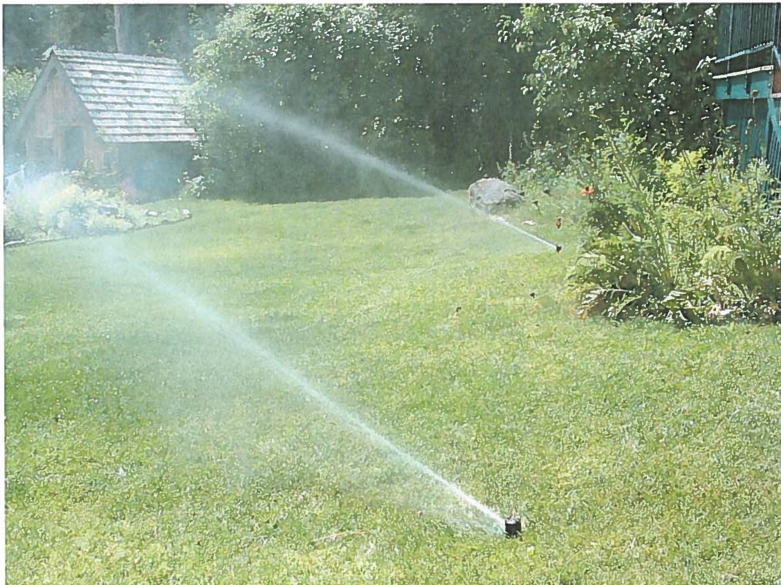
Sprinklers operating for irrigation of landscape located between house (right) and beach (left)
