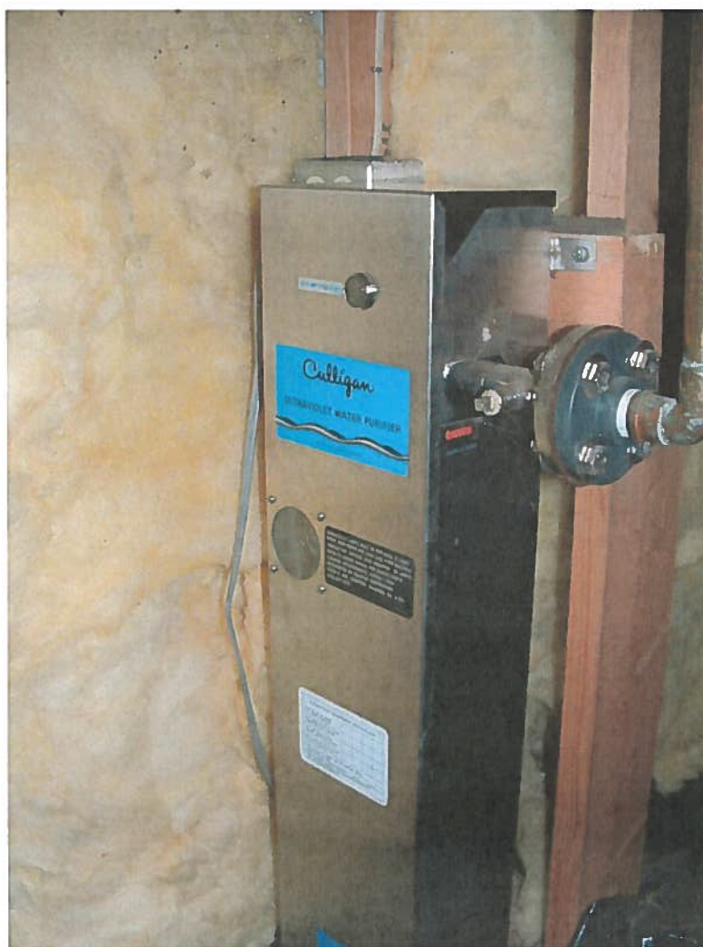
Ultraviolet water treatment.
