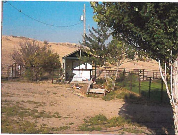
Looking west from irrigation POD well head, domestic well is located in pump house in center of photo.
