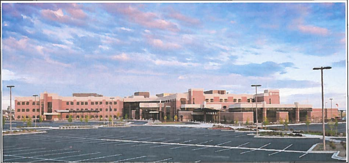
Figure 3: St Luke's Magic Valley Hospital (place of use, photo from hospital web site).
