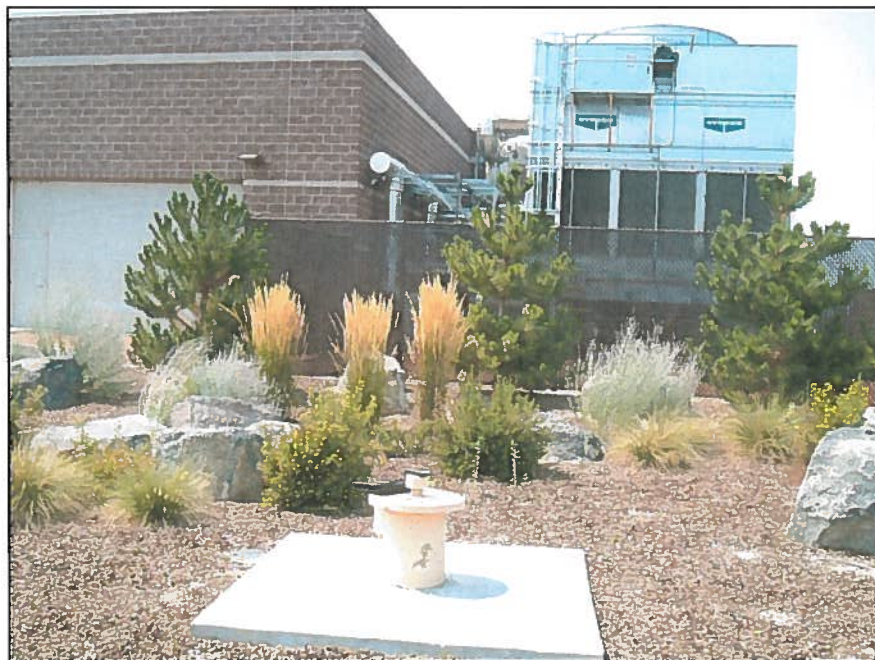
Figure 1: Point of diversion with operations building.
