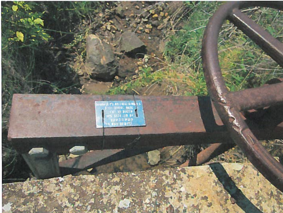
This photo shows ID tag A0016969, placed on the head gate.
