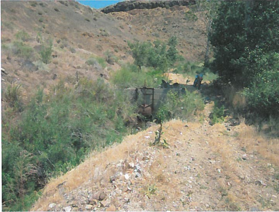
This photo shows the head gate to the canal.
