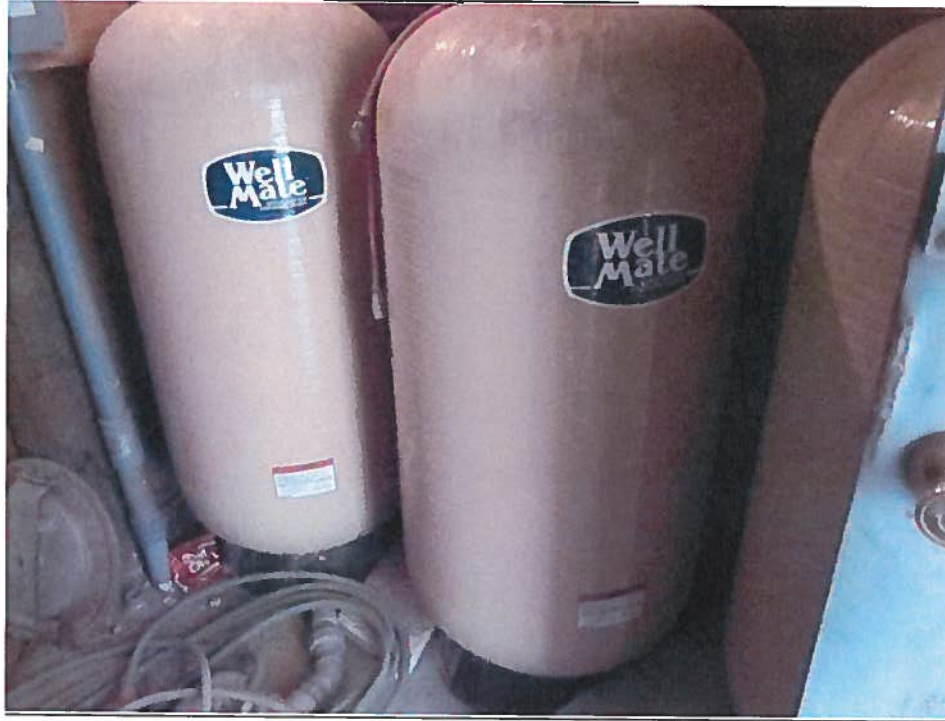
Picture of pressure tanks
