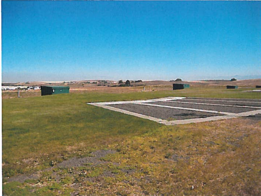
Looking at POV facing NE direction
