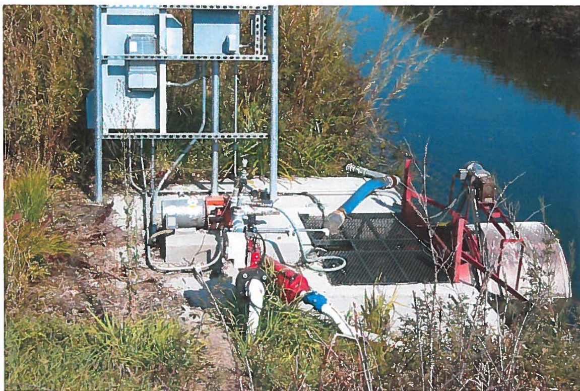
Diversion on Canal for Irrigation of church grounds
