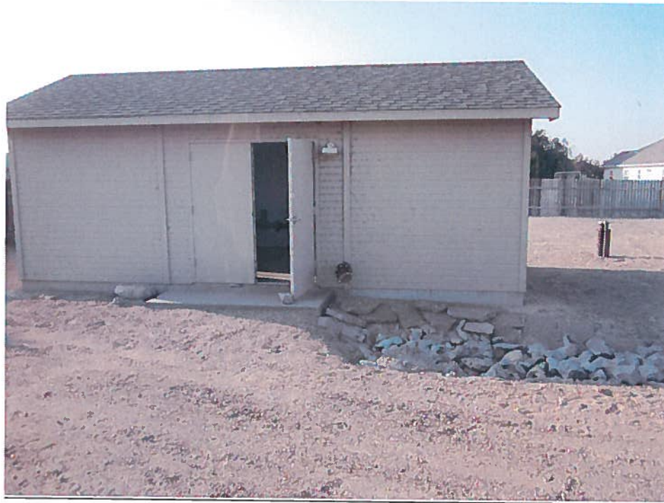
Picture of Well House
