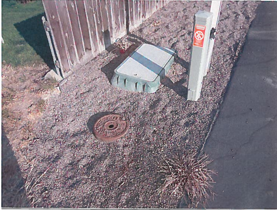
Picture of typical irrigation backflow prevention system for a lot.
