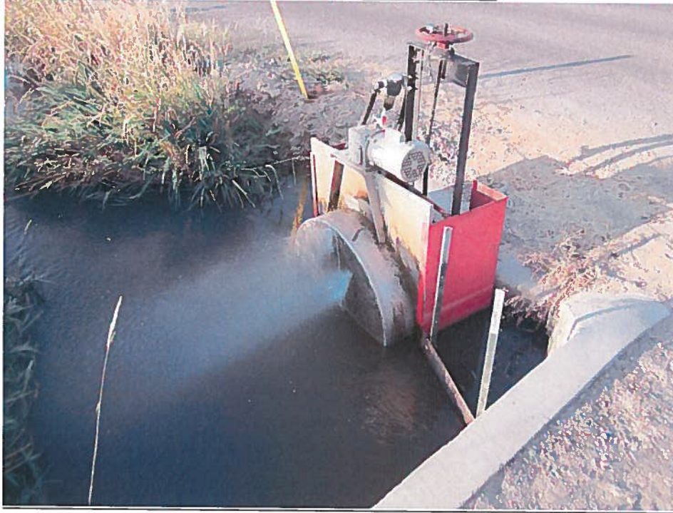
Picture of Canal Diversion Works
