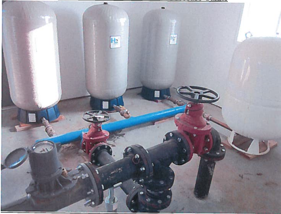
Picture inside Well House of Pressure Tanks
