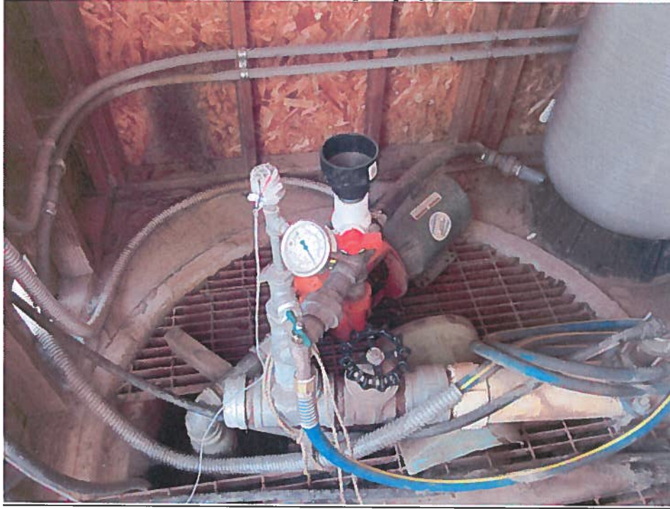
Picture of canal pump system
