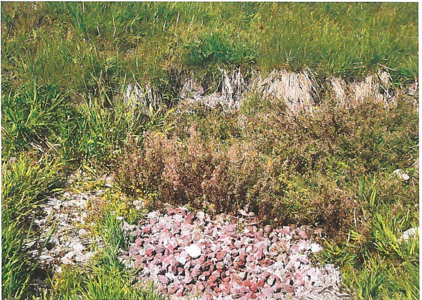
POD-Steel cistern in gravel
