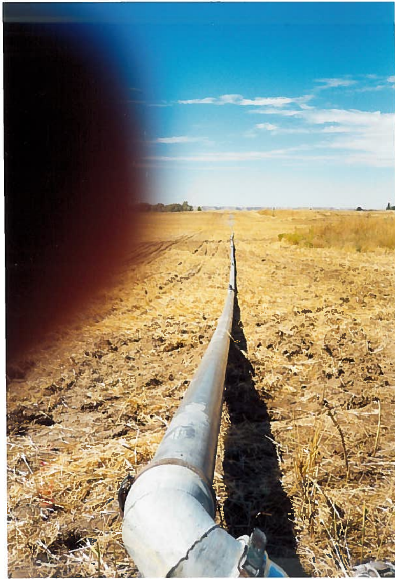
Mainline Running West From Pivot Center
