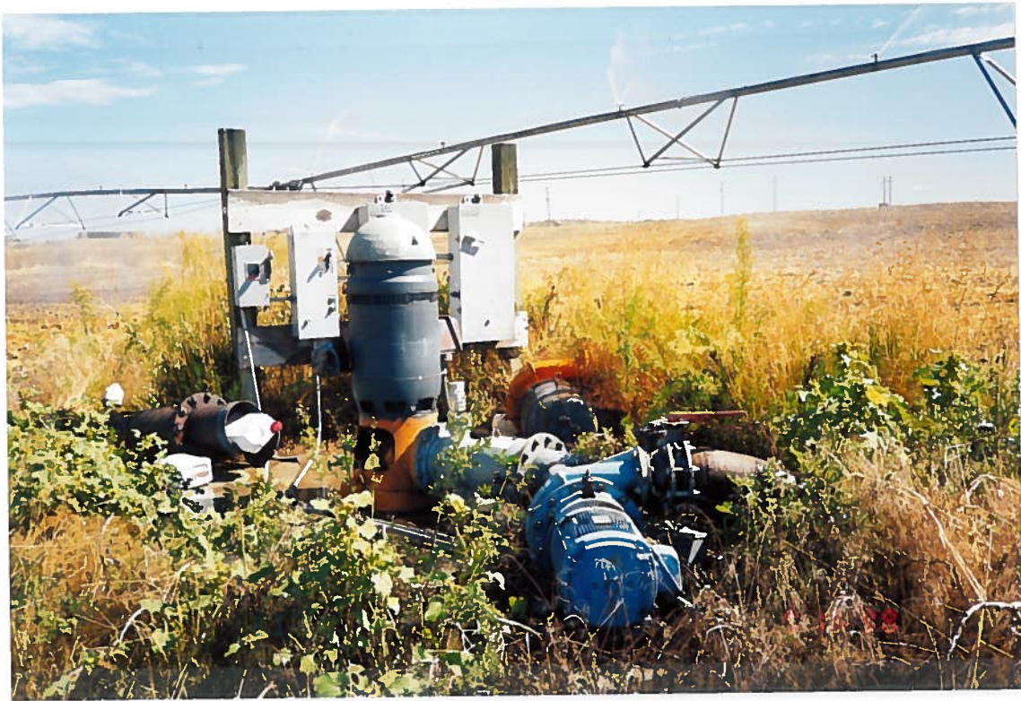
Well, Motor, Pump, Booster
