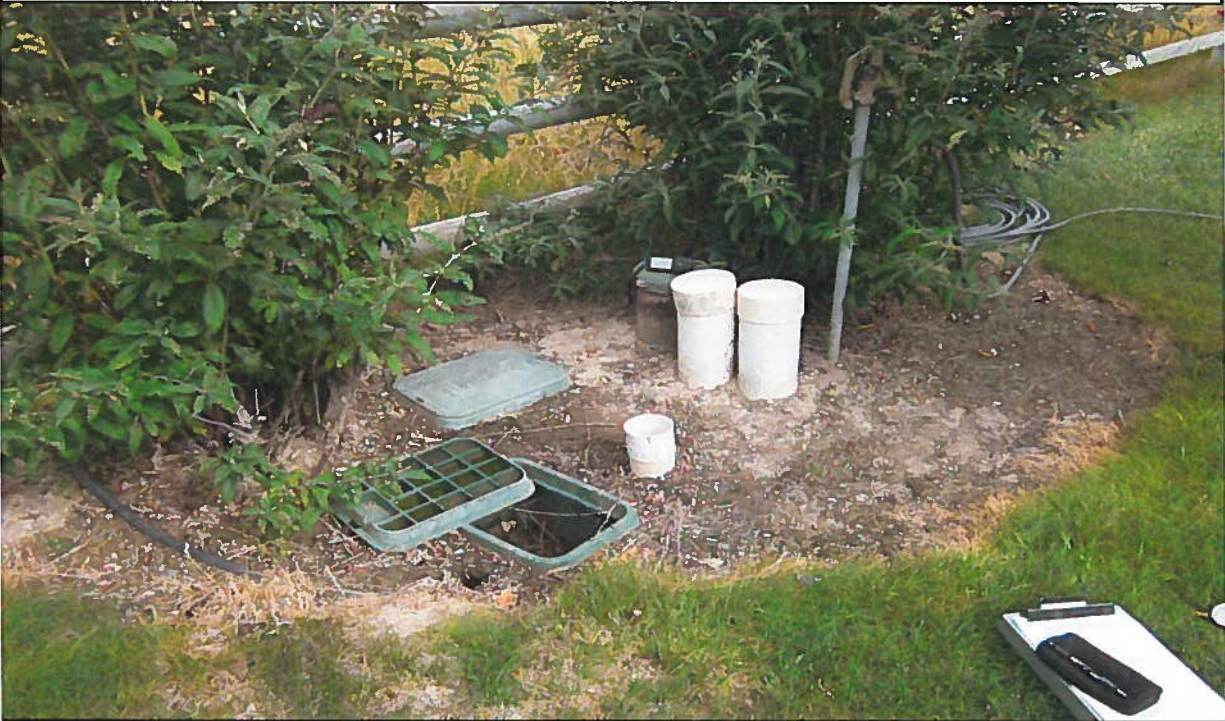
Point of Diversion: View northwesterly of domestic and irrigation well located next to fence separating the lawn area and pasture.
