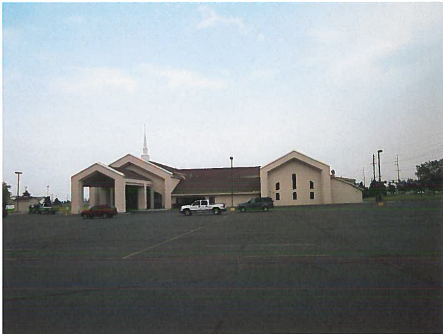
Figure 4: Church exterior. New addition (part with steeple on the left) does not use the low temp geothermal water for heating
