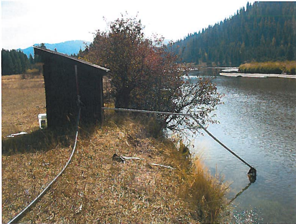
65-13914 Exam 10/9/2012: P/D pump house and 1.5 in discharge line facing south.
