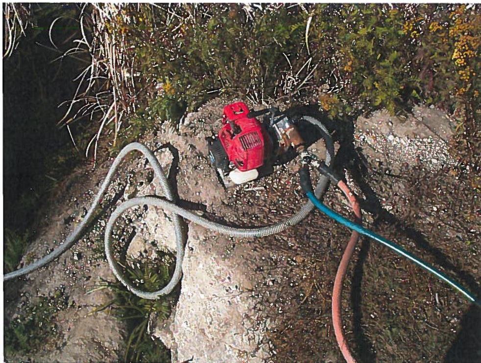
65-13962 Exam 10/9/2012: P/D pump. 1 in diameter suction hose through pump split into 2 connections for 2 garden hoses for sprinklers.
