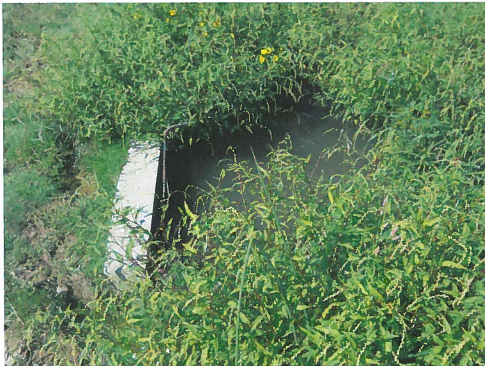
Photo of the gate into the ditch.
