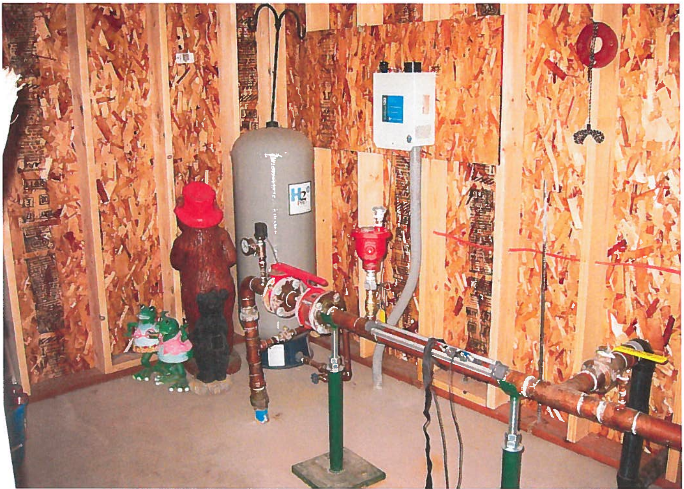
Inside of well house
