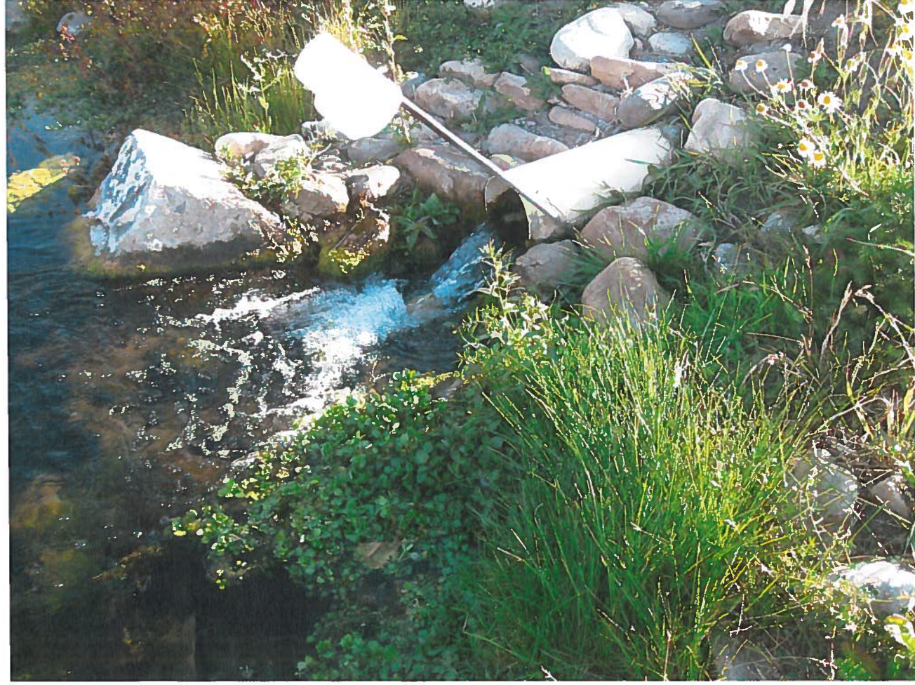
Pipe from tile drain system
