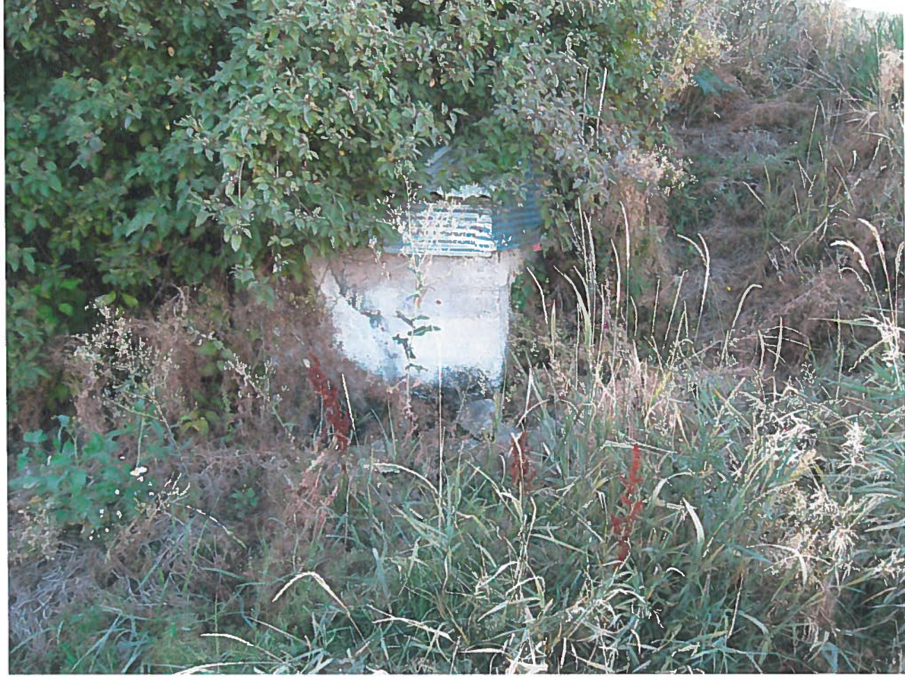
Spring box for domestic spring
