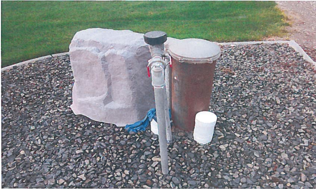
Well adjacent to the private road off Stamm Lane. Well is on the Corisis lot, middle lot of the 3 lots served by this well.
