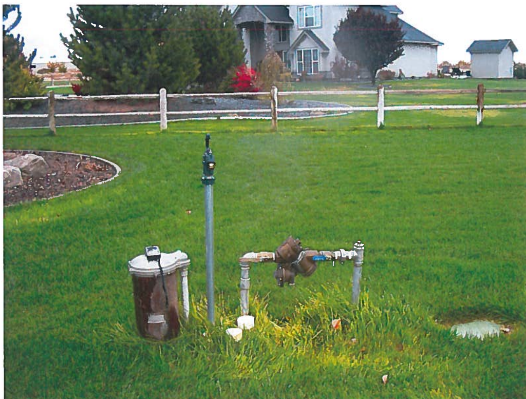
63-33088 Exam 10/22/2012: P/D well and portion of lawn P/U, neighbor's home in background.
