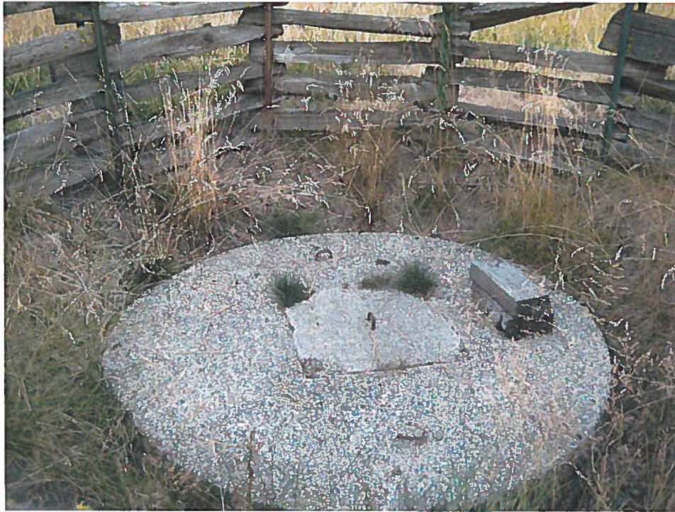
Spring box 1,000 gallon capacity
