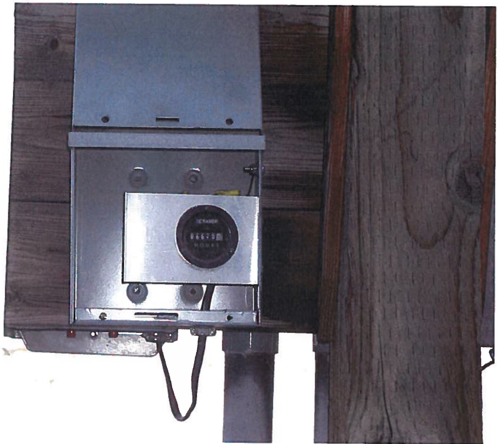
Elapsed Time Meter (Units in hours) for Williams Lake Recreational Water & Sewer District for water rights 75-7589 & 75-7590.
