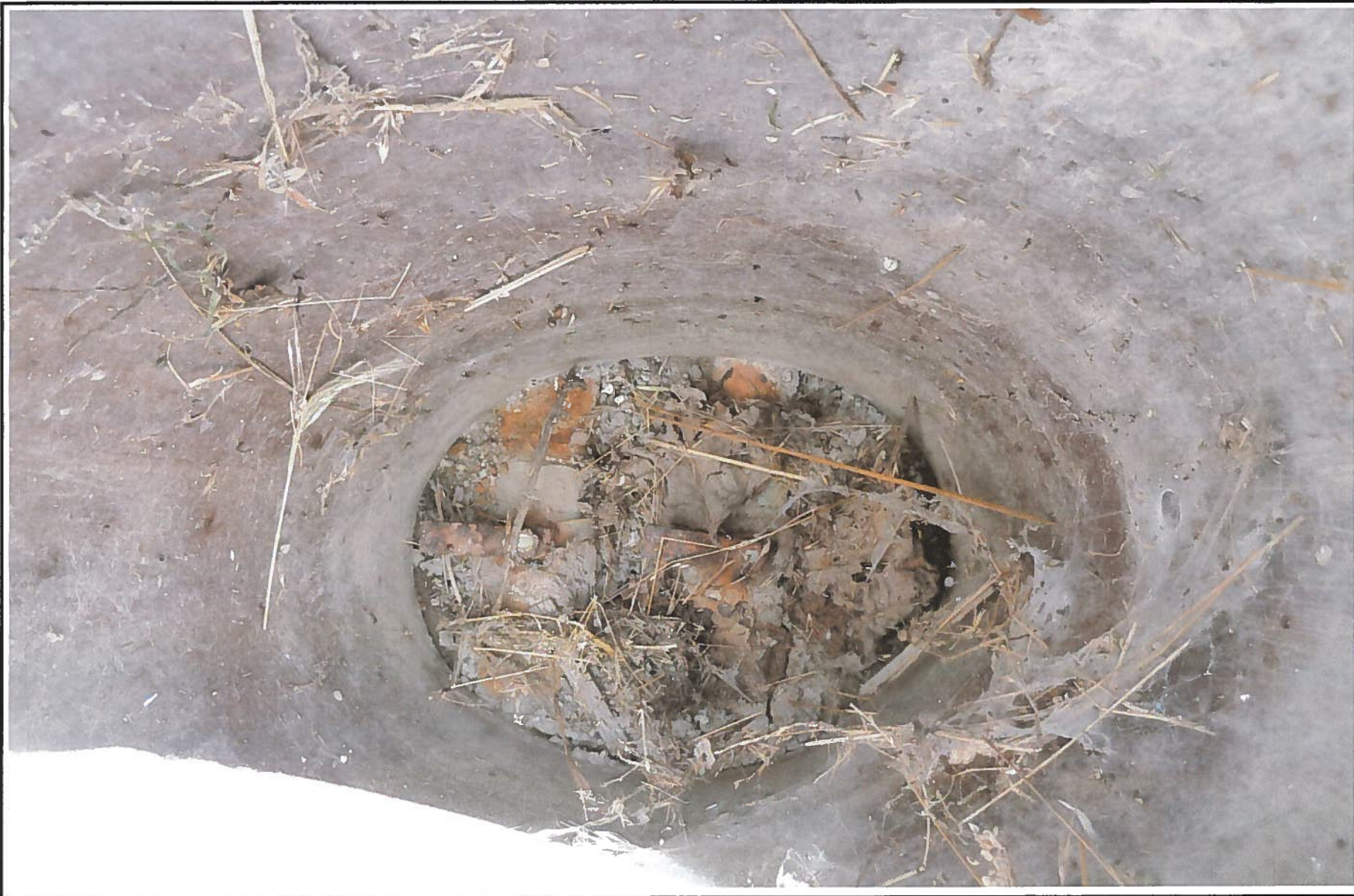
FIGURE 9: IRRIGATION SYSTEM VALVES RUSSELL THOMPSON PERMIT NOS. 47-7578 AND 47-7579 SITE VISIT ON 6/8/2012
