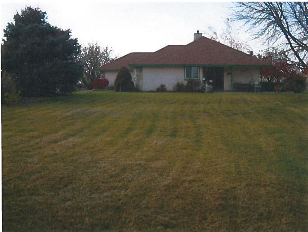
63-12115 Exam 11/8/2012: Portion of P/U (Lot 2) from outside pump house/shed facing west.
