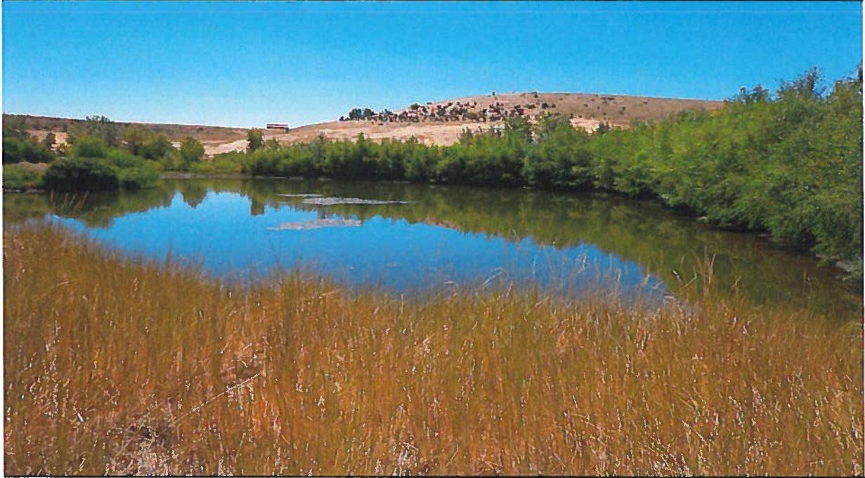
Point of Diversion/Place of Use: View southeasterly of wildlife storage pond. Dam with a thick cover of trees and brush is shown on the south and west end of the pond.
